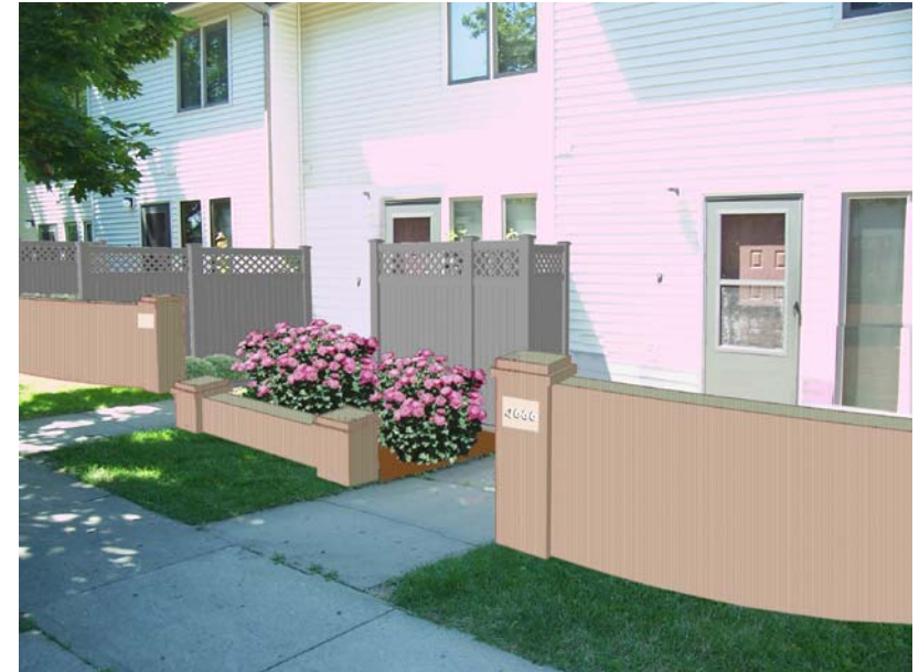
POURED CONCRETE WALL
